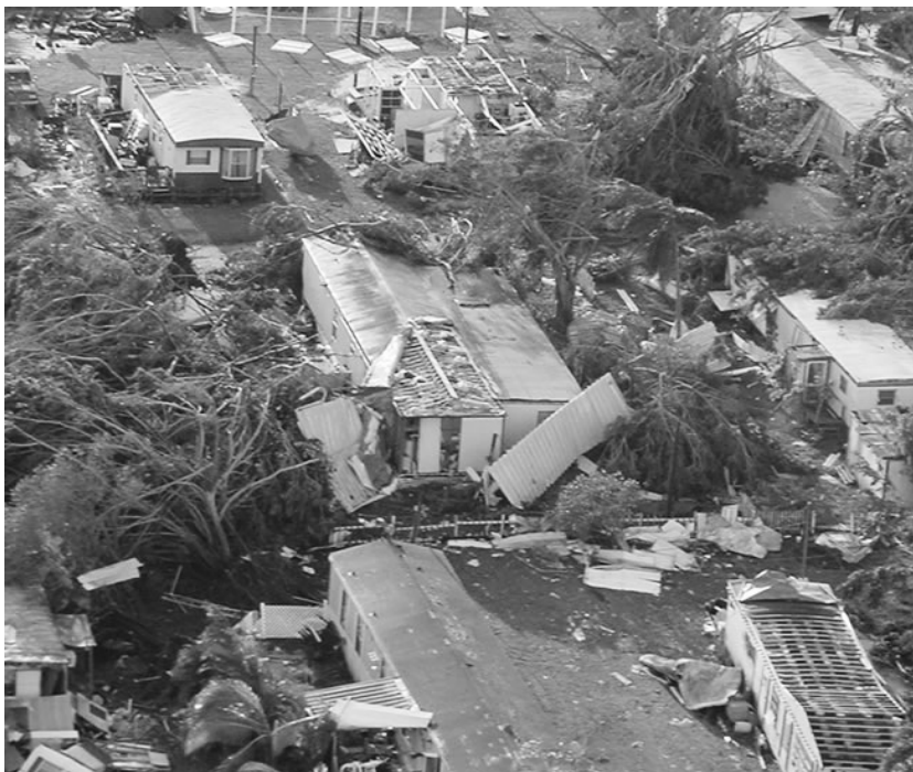
Hurricane Charley devastated the Pink Citrus Mobile Home Park in the Bokeelia area of Pine Island.
