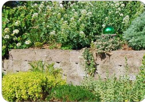
Retaining walls can be an effective solution to create level areas for planting while protecting steep soil excavations from erosion.
