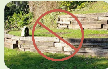
WOOD RETAINING WALLS
