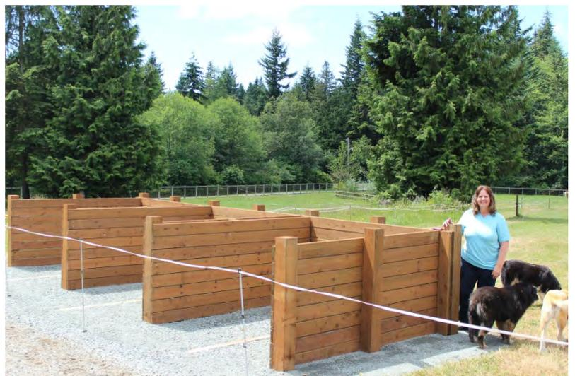
Both bins have a 5/8" minus compacted gravel base, typically 6 – 8" thick, using gravel that is a Washington DOT specification. Down the middle of each bin is an 'I' beam which prevents a tractor loader from scraping up gravel when the bin is being emptied. Landowners can also choose a concrete base, with or without curbs. A roof can be added as well. In Lyn's case, she'll likely use tarps to keep rain off the piles and prevent any runoff.
