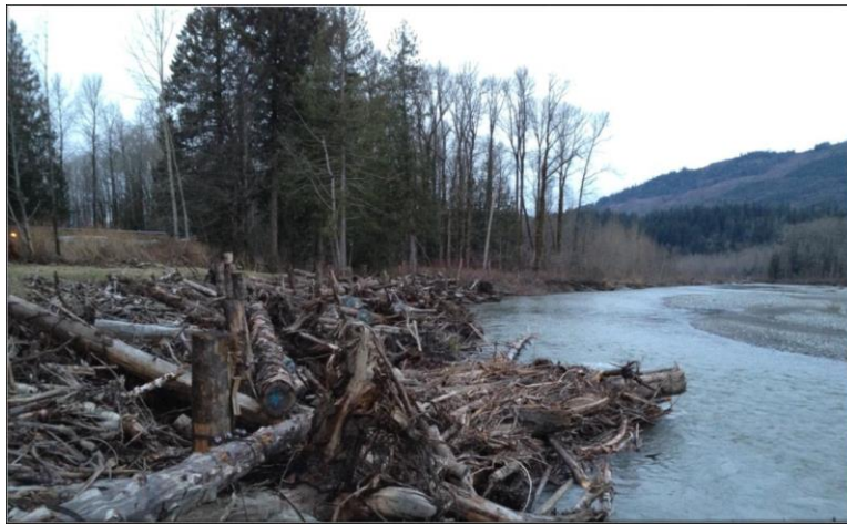
Figure 3 – Example of a large wood revetment in the South Fork Nooksack River, WA (USBR and ERDC 2016)
