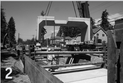
A stormwater vault is being assembled in the trench shown in Photo 1.
