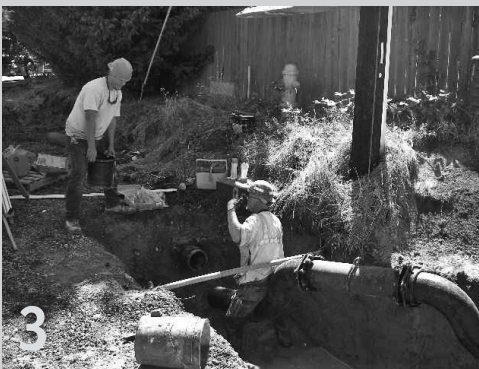
The crew spent a lot of time in small and large trenches working on the drainage system and utility lines.
