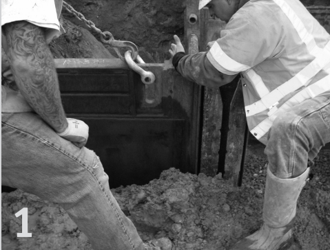
Temporary metal walls kept two large trenches from caving in during construction.
