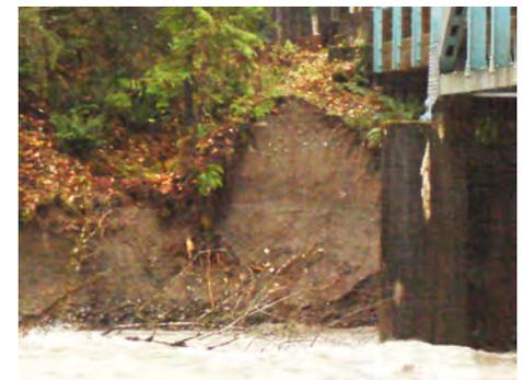
*Erosion of upstream bank on east side*
