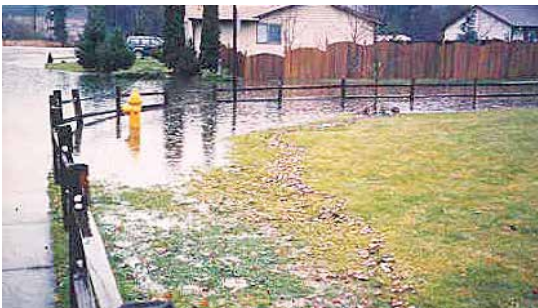
An undersized culvert led to flooding in Marysville in 2005.
