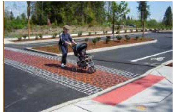
*Mid-block crosswalks were elevated approximately 6 inches above the traffic lane and installed at several locations along the new road. Pedestrians are more visible to drivers and drivers must slow down to traverse these raised crosswalks.*
