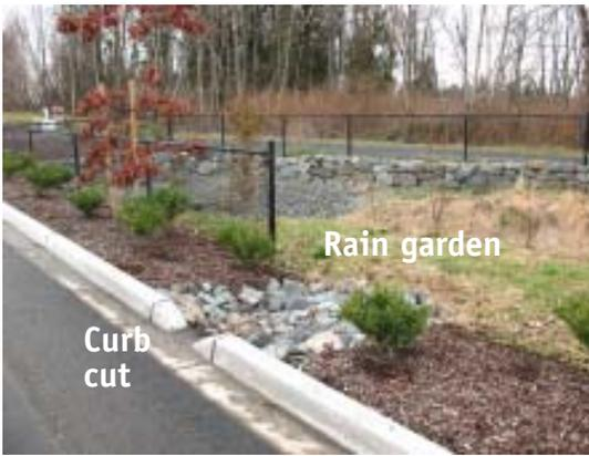
*Cuts in the roadway curblines allow water to spread out evenly as it flows through the rain gardens and eliminates maintenance of catch basins.*
