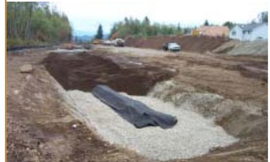
*Shaping underdrain material & soil mixture*
