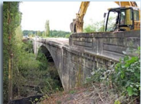
*The cellular concrete used was Elastizell. It is produced by mixing an expansion material to a cement mixture. The result is a low-density (load-reducing) material used as fill for applications such as behind retaining walls, at bridge approaches, over culverts, under roadways and over poor soils. The density ranges from 30 to 110 pcf; Normal compression strength can range from 140 to 2400 psi, depending on what is required for the application.*
