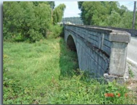
Square footage of the bridge deck was increased by 62% without adding weight. By using the existing concrete arches, engineers designed a wider two-lane bridge deck, eliminated the need for a complete bridge replacement, and shortened the project by 4.5 years.
