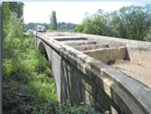
engineers needed to find a way to reduce weight somewhere else. They studied several light-weight materials to replace the existing heavier soil fill in the arches.
